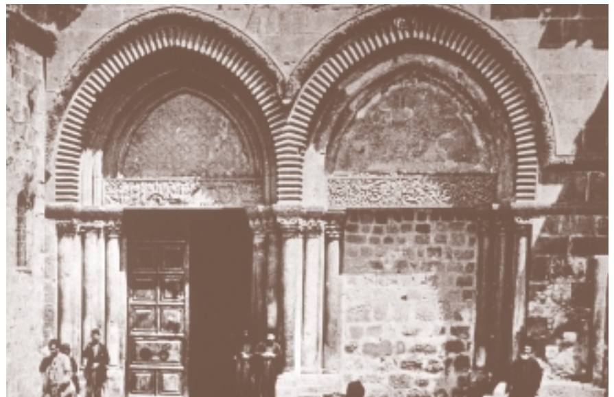
Figure 4: Jerusalem, the Holy Sepulcher, south façade, doors and windows adorned with cushion voussoir.
