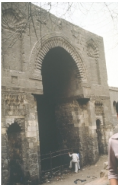
Figure 5: Cairo, the Great Mosque of Baybars (1267–1269): Central portal adorned with cushion voussoir.
